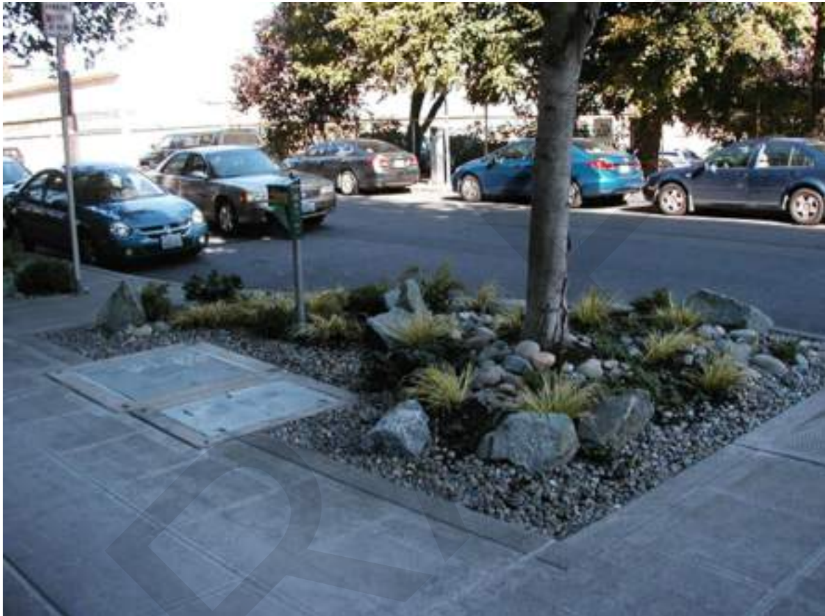
Rocked pet potty area that is connected to sanitary sewer.
